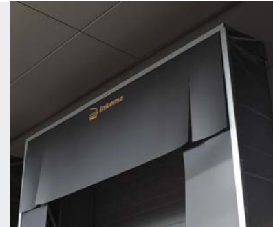
Shelter with 10% slope for draining water.
